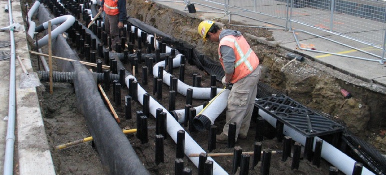
Suspended pavement systems allow roots to thrive, growing large, healthy trees, while also storing overflow stormwater. Photo above shows a Silva Cell™ System being installed in Toronto, Canada 2010 (Deeproot.com)
